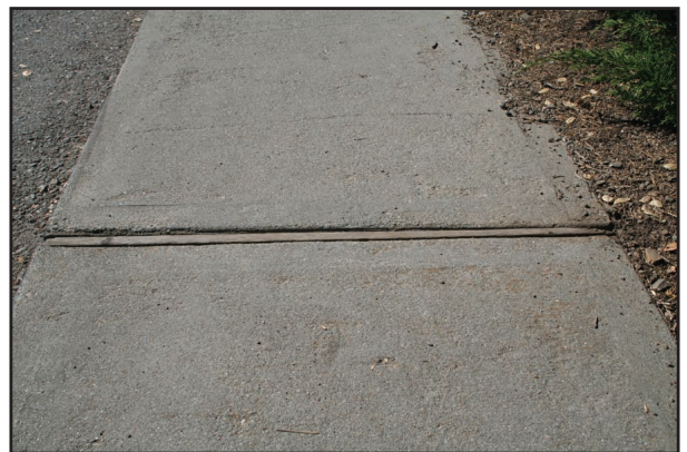
Compressible concrete joint
