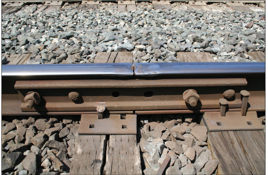
Train track expansion joint
